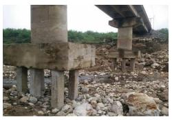
b) Erosion of bridge pier foundation in Ky Anh - Ha Tinh
