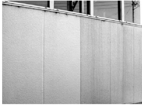
Figure 4. Treating the surface with the coating does not change the appearance of the surface; however, the self-cleaning phenomenon will result in the surface staying clean for 3 years or more [Bio Pro Coatings]
